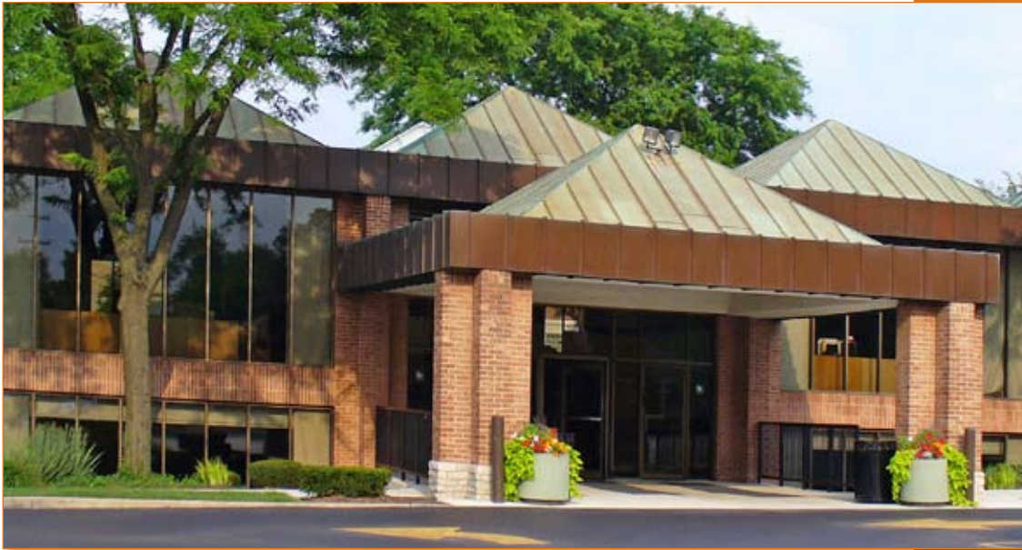
Harris Bank, Hinsdale, Illinois John A. Mayes, Donald H. Williams & Partners/ Architects A.I.A. R. H. Roberts Construction Co., Builder Roof installed 1969
